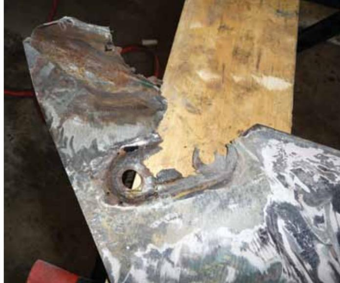
Rusty floor pan... holes and rusted out flange running the entire length of the side of the floor pan
